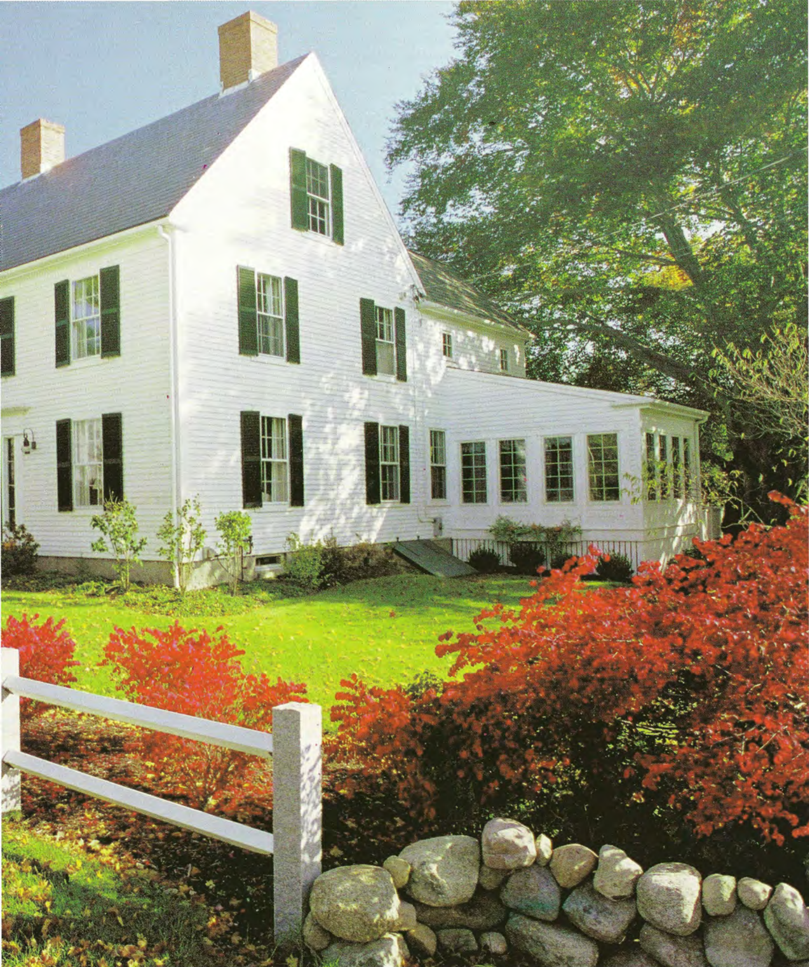
The front of this 1840's farmhouse was fully restored to its original while the rear wing was almost completely demolished, redesigned and expanded. The enclosed porch is completely new, designed to snuggle up under the cool shade of the tree. The barn had a small addition with the contemporary garage added. (Left) The semicircular master bedroom balcony deck sits on the porch roof looking across the bay.
